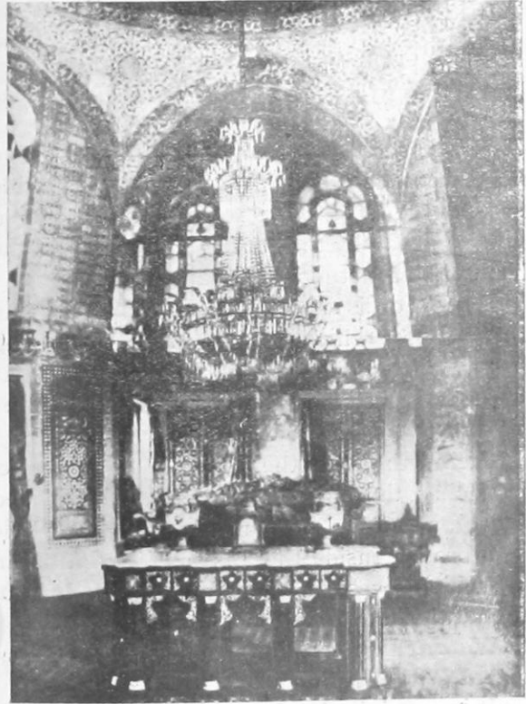
Interior view of the Bagdad Kiosk
