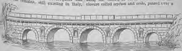
Bridge at Ariminum.
