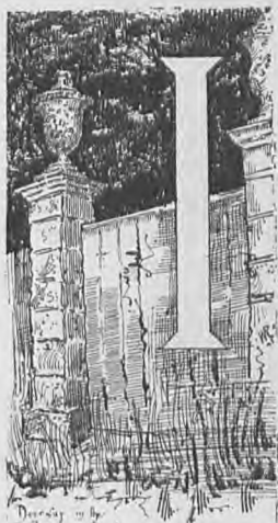
Carriage Entrance, within second Lodge Gate.
