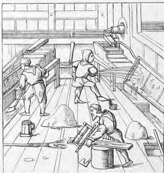
Fig. 154. "The Rack." (Agricola.)
